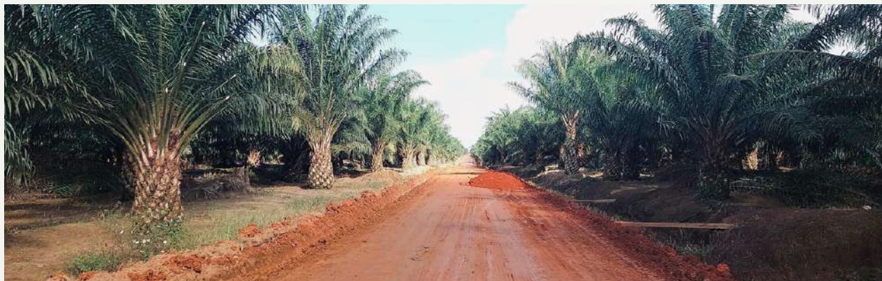
Pembangunan akses jalan penghubung antar kampung Concession Construction of access roads between villages
